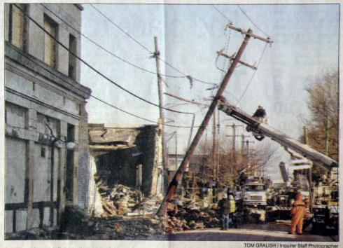
A utility pole was left testering yesterday morning when the wall of a building collapsed on Fourth Street just north of Vine Street, spilling brickwork and other debris into the pole and across the road. Workers had been dismantling the building as part of a project to turn the eight-story building at left into condominiums. No one was injured.  During demolition
