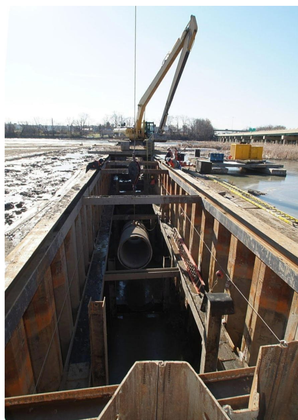
Sixty feet long cofferdam segment with 54 inch diameter pipe installed
