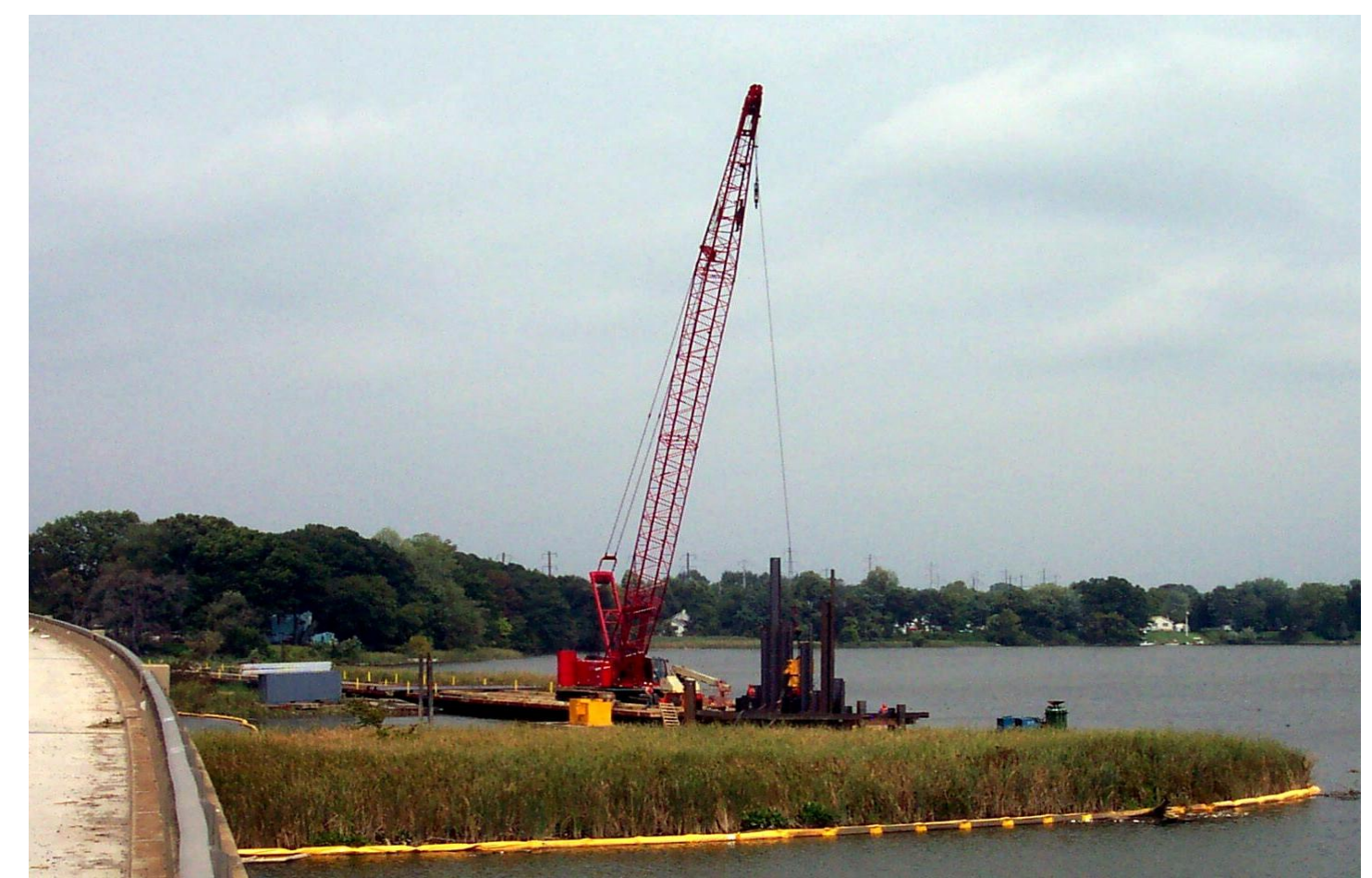
Phase 1 SSP installation from the north shore
