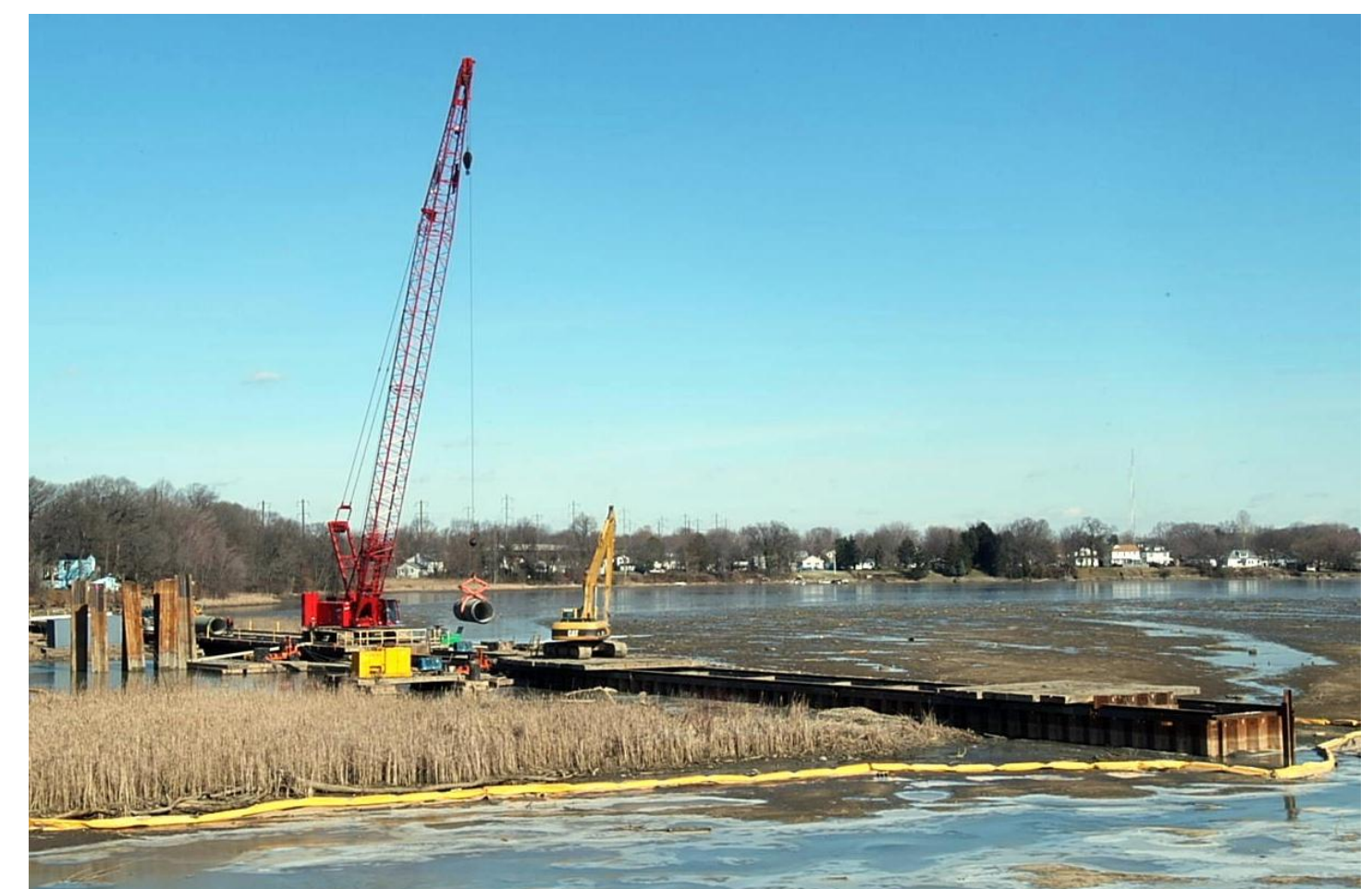
Phase 1, north shore 20 feet long initial cofferdam with pipe installation
