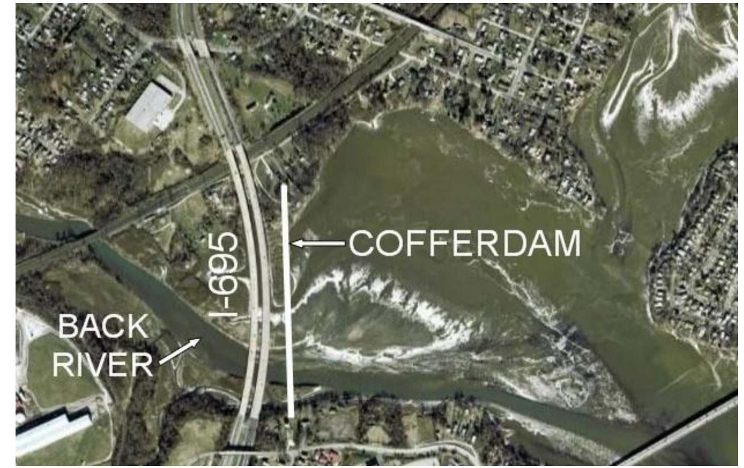
Aerial view of river crossing, east of I-695 bridge.
